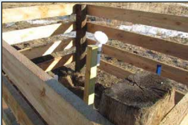
Examples of satellite unit installations in a pasture location
