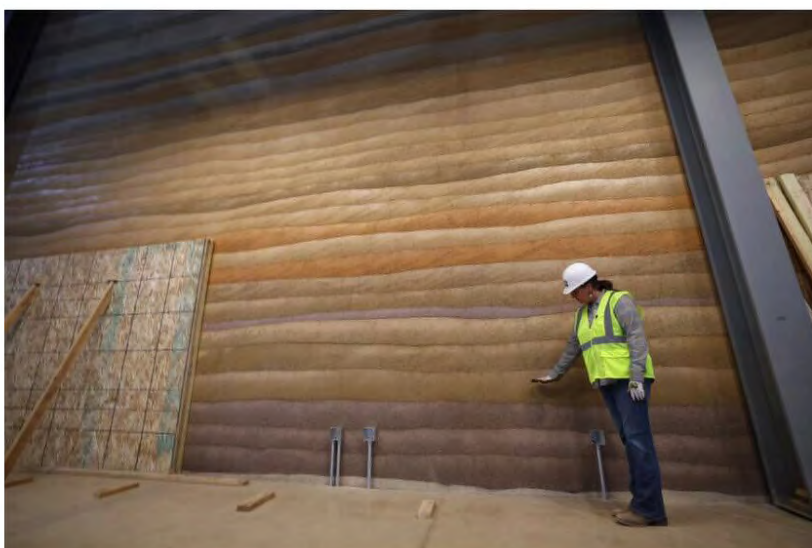
Jenn Carroll, manager of sustainability for the Theodore Roosevelt Presidential Library Foundation, points out the layers of a rammed-earth wall installed inside the library Tuesday, May 27, 2025, near Medora.
