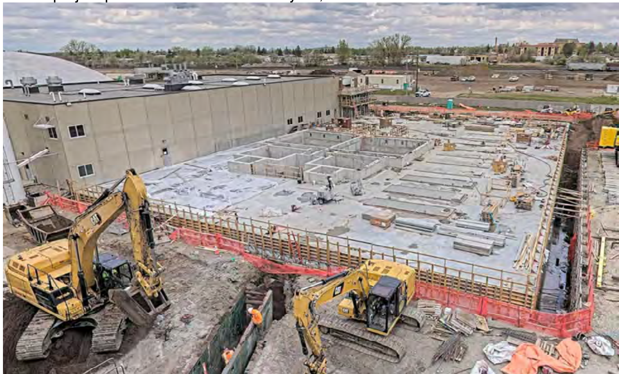
SWTP project picture below taken on May 21, 2026
