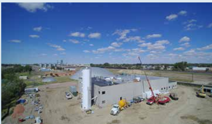
Construction of the Southwest WTP
