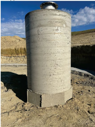
Inlet pipe encasement
