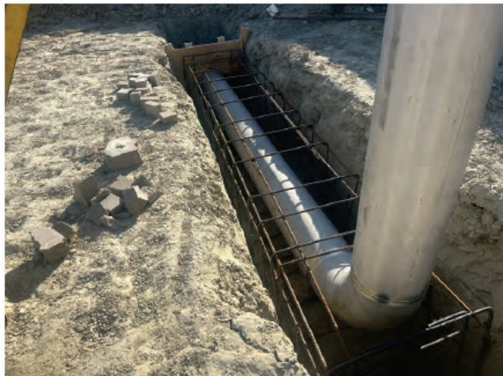
Outlet pipe size 4 rebar
